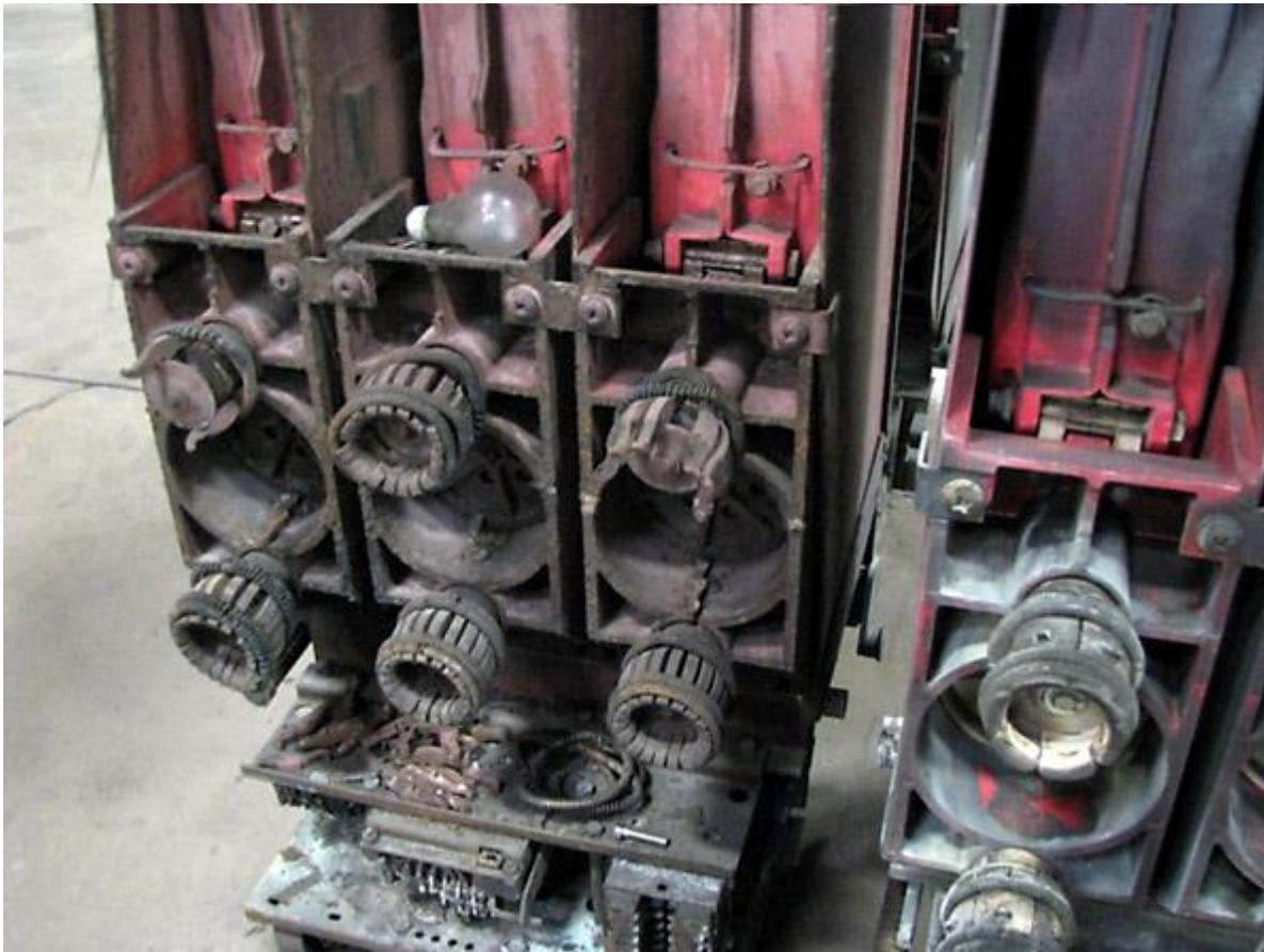
**Photo 2. An unmaintained circuit breaker is a bomb waiting to explode.**
